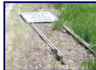
Figure 6. Typical Roadside Signage
